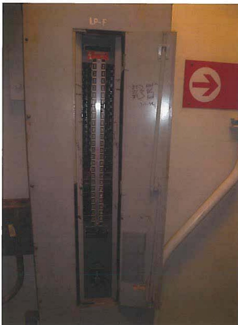
EXISTING PANEL "LP-F"
